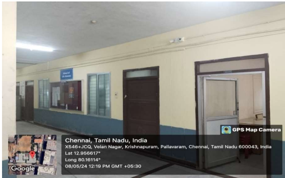
CCTV in all corridor
